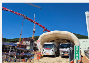
Inflatable Noise barrier for concrete pump trucks
