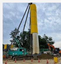
Sound-absorbing pads for pile drivers
