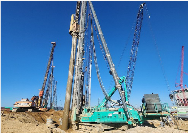
Pile driver concentrated water spraying system
