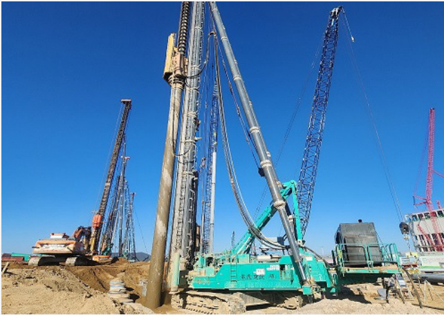
Pile driver concentrated water spraying system
