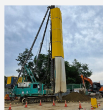
Sound-absorbing pads for pile drivers
