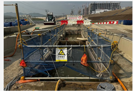
Wheel-washing water reuse facility
