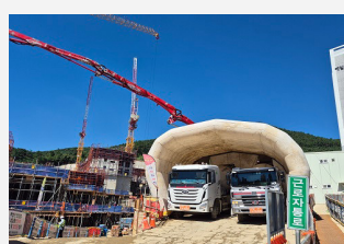
Noise barrier inflatable for concrete pump trucks
