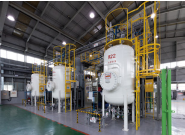
Refrigerant Recycling and Purification Facility
