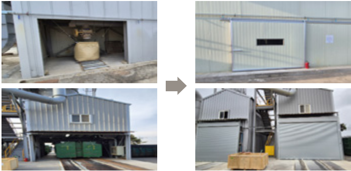
Dust Dispersion Prevention Doors for Dust Collection Equipment
